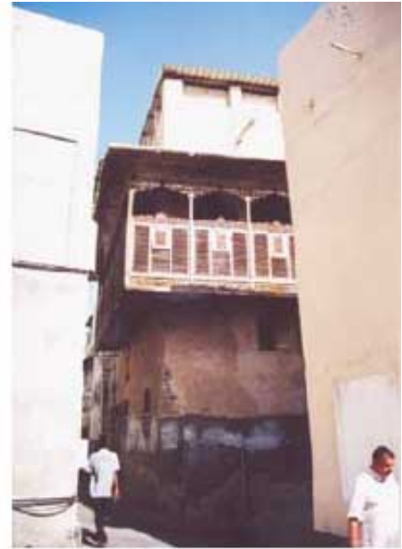
2.2 - AN EXAMPLE FROM MANAMA, ALSO SHOWING THE CHAMFERED CORNER AT THE JUNCTION OF TWO STREETS, 2006.
