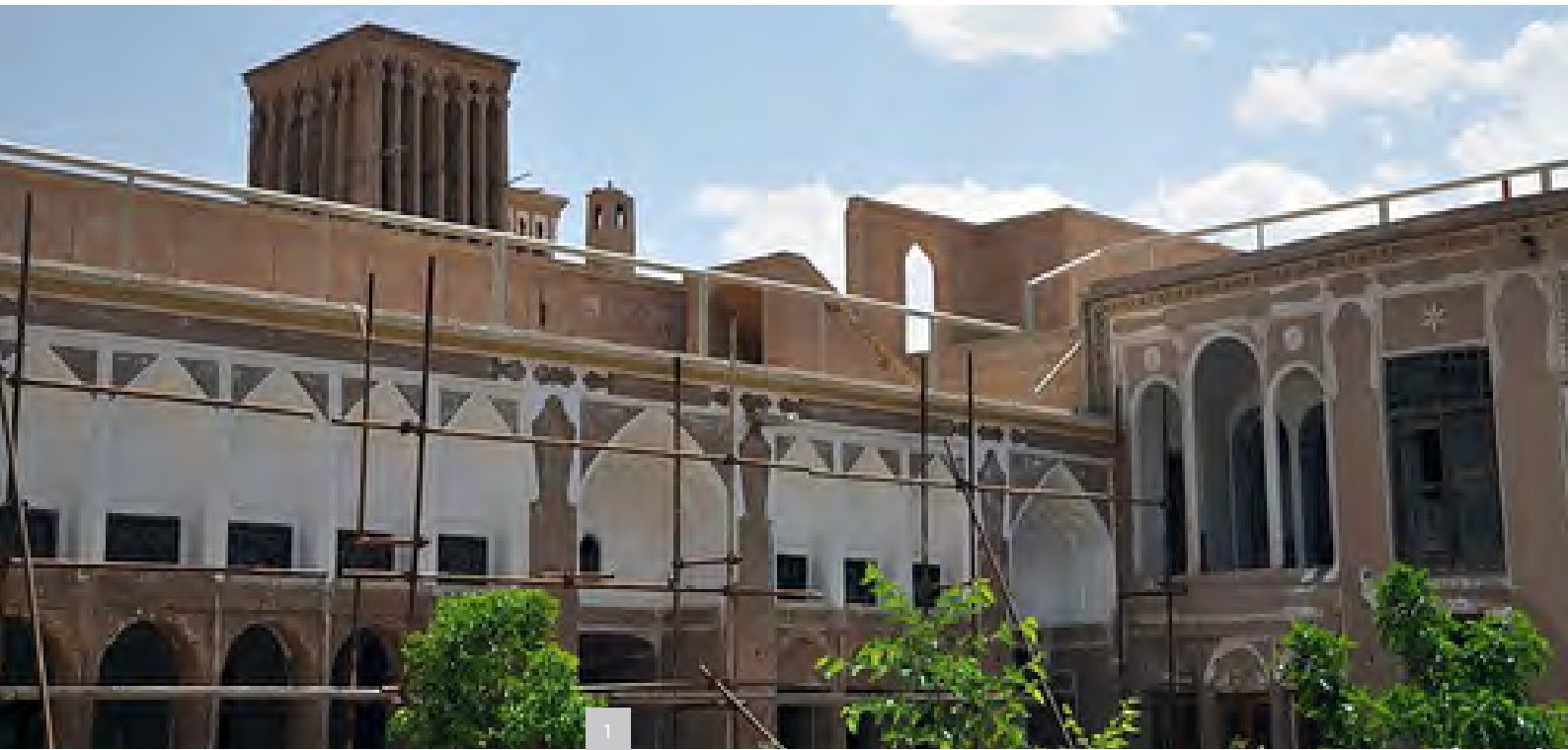
Images 1 & 2- Iqbal factory during renovation
