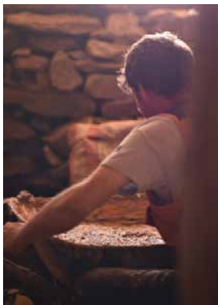
Figure 8 Skilled construction worker mixing traditional materials "Lokh" with clay and water to smoothen walls.
