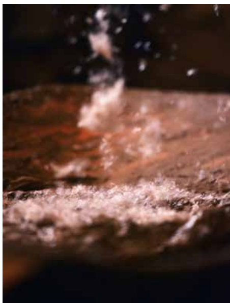
Figure 7 Traditional wild flower "Lokh" being added to the mixture and used in the final steps of construction to smoothen walls.
